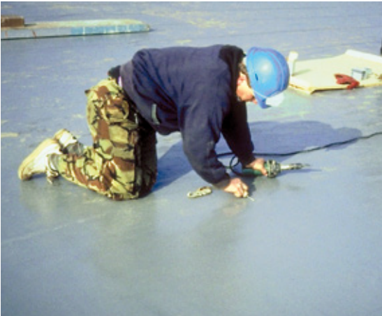
fig. 2: Verification of weld security
